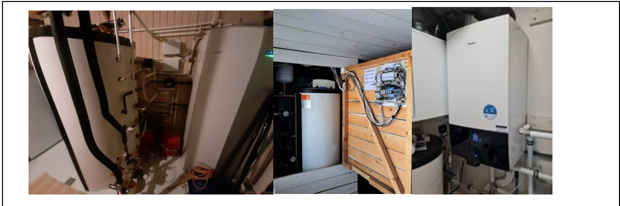
Figure 4.7: Examples of Estonian residential flexible resources – ground source heat pump, heat exchanger, air-water heat pump
